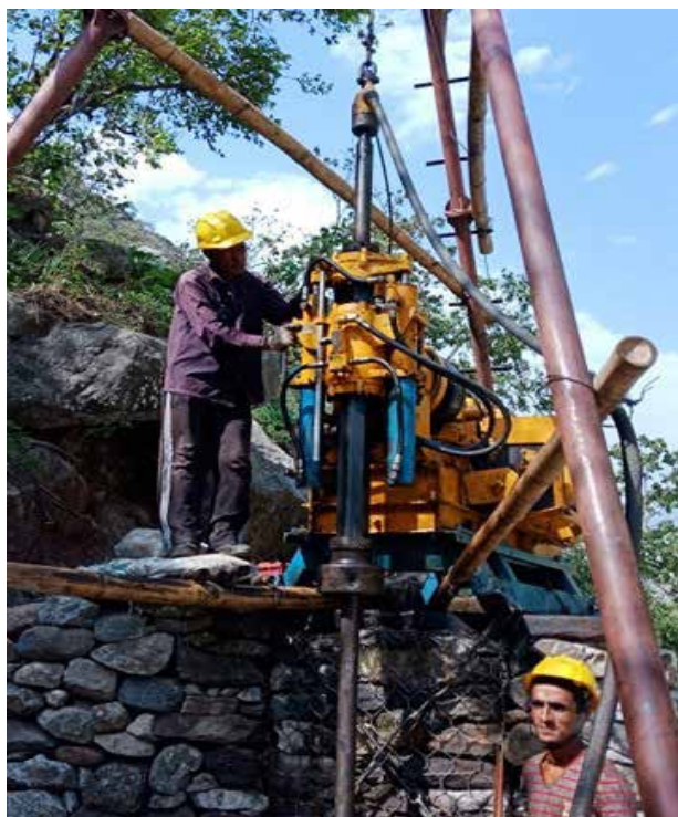
Core Drilling works at Phukot Karnali HEP
