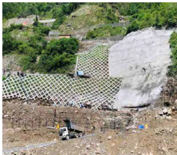
Powerhouse Slope Support
