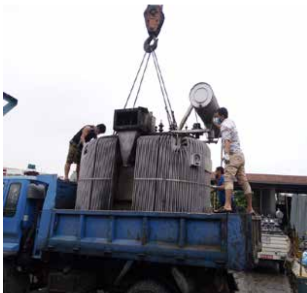
Power Transformer Unloading
