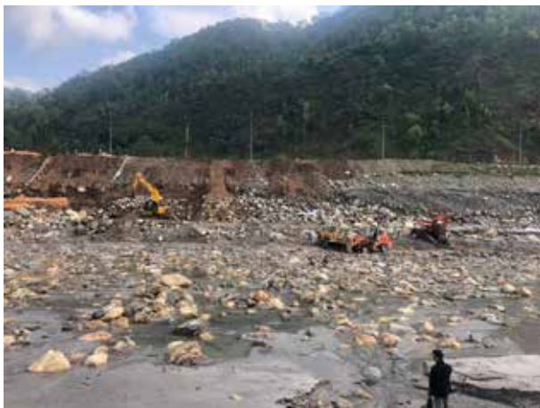
Repair and Maintenance work of Rip Rap of Desander Basin
