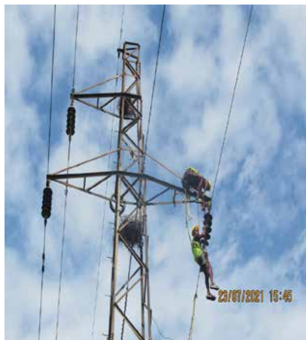
New Conductor Stringing Works
