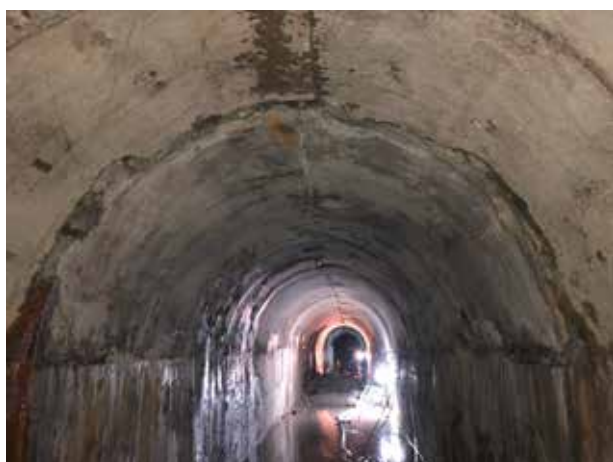
SUHEP's completed Tunnel Lining
