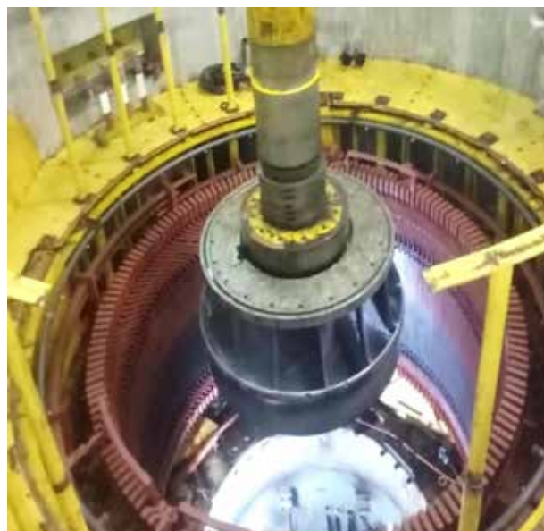
Dismantling of Runner for its Replacement.
