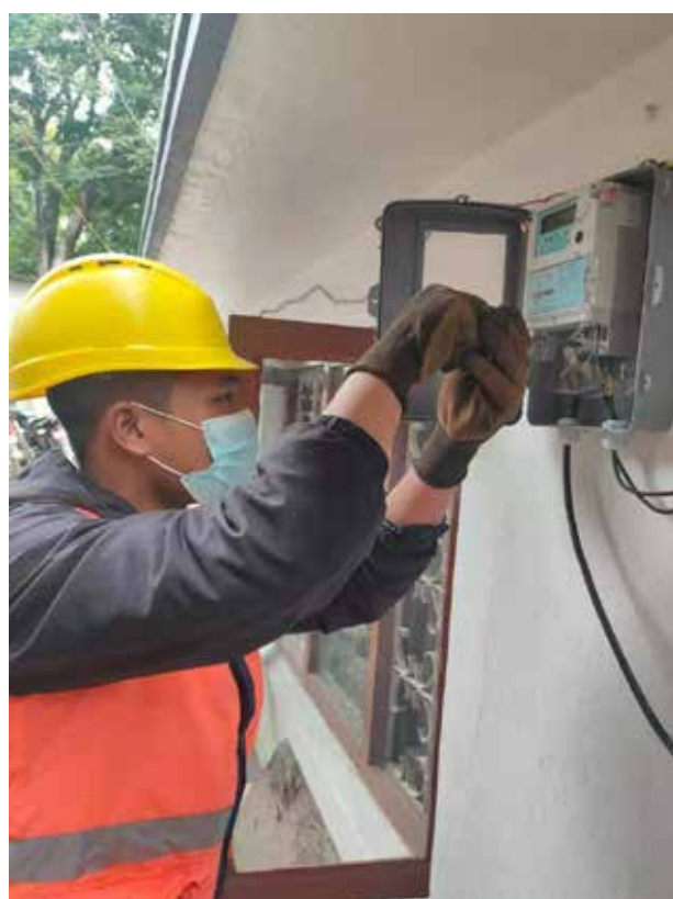
Smart meter being installed
