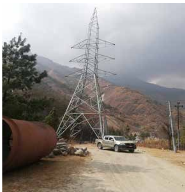
Erected Tower for Power Transmission
