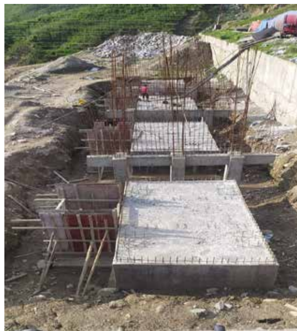
Transformer foundation works under progress at Bahrabise Substation
