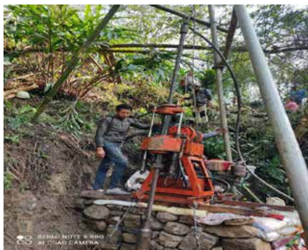
Borehole Drilling at nearby Proposed Powerhouse Site
