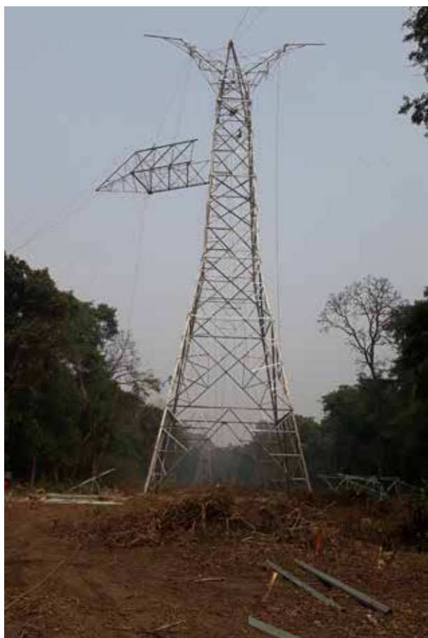
400 kV Tower Erection Works
