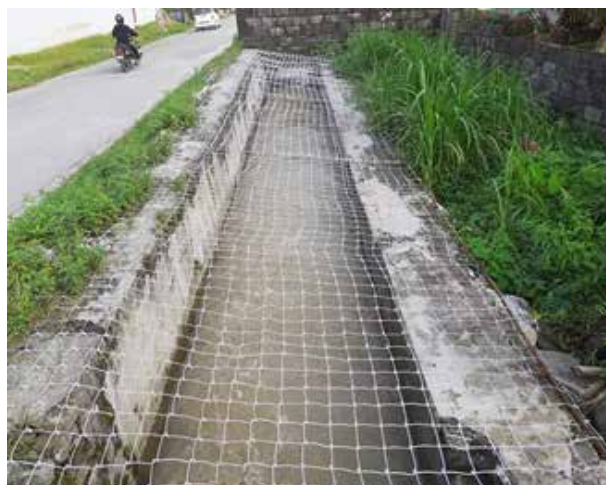
Repair and maintenance of power canal with protection mesh wire.
