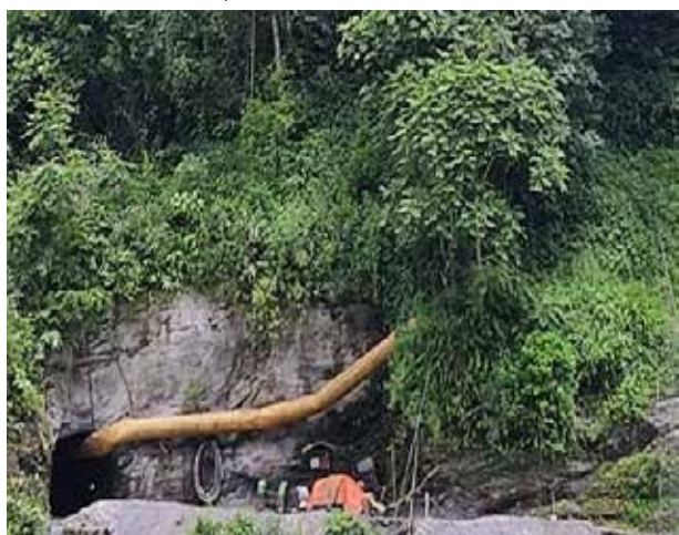
Test Adit at Proposed Powerhouse Site
