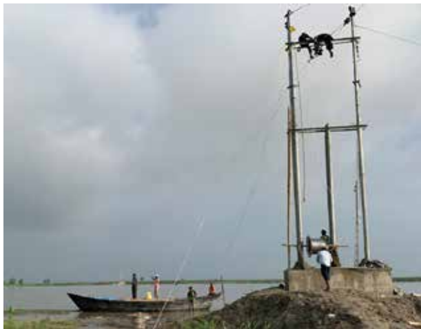
Construction works for stringing conductor across Koshi River for Rural Electrification at Hanuman Nagar Kankalini Municipality-13, Gobhargadha.
