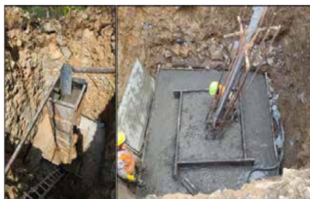
Concreting Works in Tower Foundation
