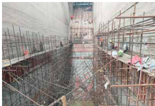
Rehabilitation Work of Spillway No. 3 of Dam
