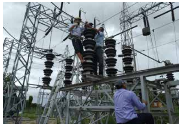
132 kV ISOLATOR REPAIR WORK
