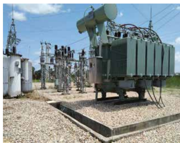
Upgradation of 33/11 kV, 10/13.3/16.6 MVA Mainapokhar Substation, Gulariya
