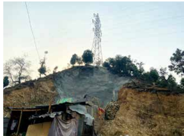
132 kV 110 no. tower protection work
