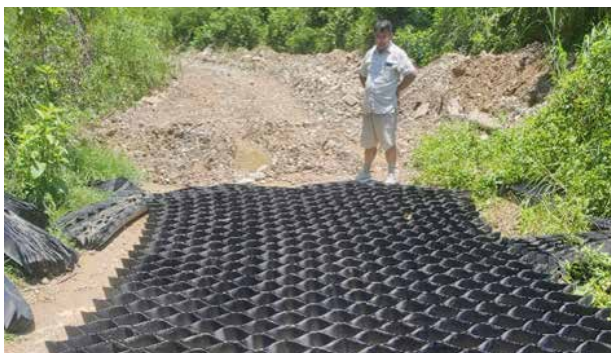
Surge tank road repair by using GEOCELL
