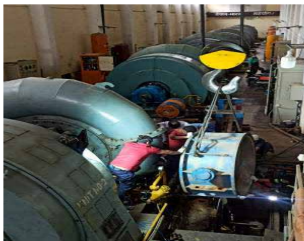
Assembling of MIV in Unit No. 2
