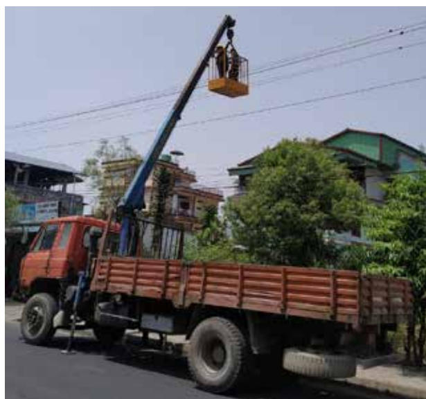
Twinning of 11 kV conductors using crane with bucket
