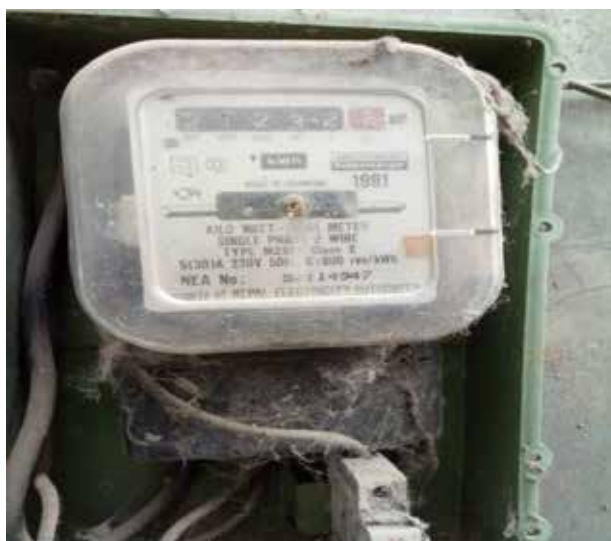
Electricity theft found by Loss Reduction Division at Dhangadi DCS (Theft is done by drilling hole in electromechanical meter)
