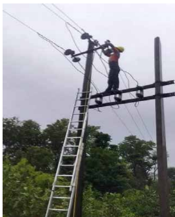
11 kV line maintenance work under Mahendranagar DC
