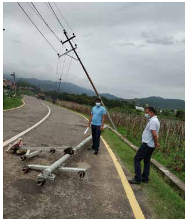
Maintenance work for inclined double feeder pole at ShreeRamPati, Panchkhal.
