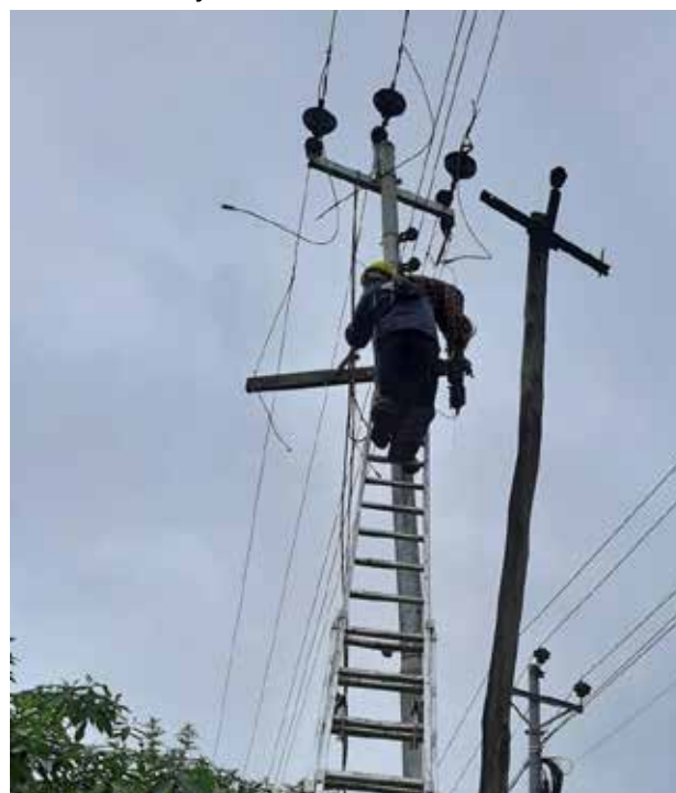
Replacement of 11 kV wooden poles by Steel Tubular Poles at Deumai, Illam
