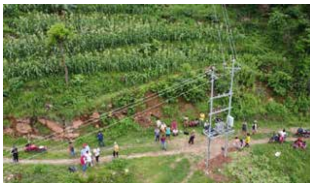
Installation of 11/0.4, 50 kVA Distribution Transformer under Solu Corridor Rural Electrification Project
