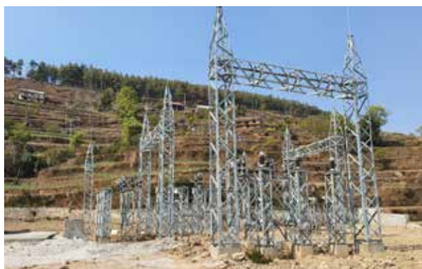
Construction of 33/11 kV, 6/8 MVA Dorambha Substation at Ramechhap
